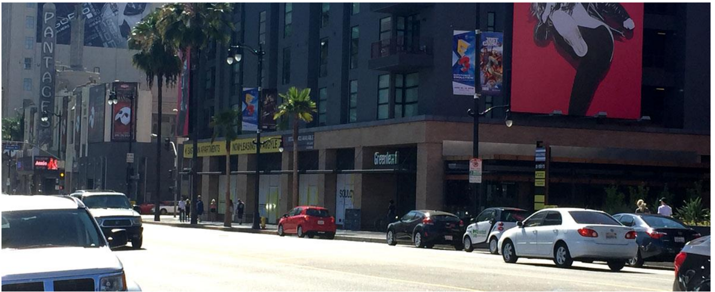
10. View looking westerly along the north side of Hollywood Boulevard.
